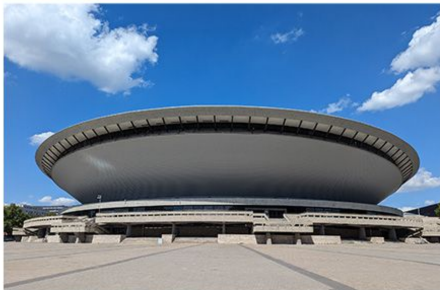
Spodek in Katowice, Poland
